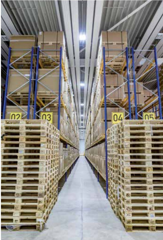
Zehnder radiant ceiling panels are operated in winter operation with a maximum flow temperature of 38°C and 30°C return temperature, which ensures optimum energy efficiency. In summer operation, the flow temperature is 16 °C and the return temperature is 18 °C. A dew point monitor was also installed for the cooling mode.
