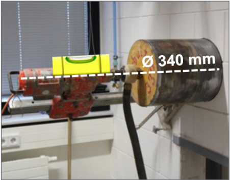
Fig. 2 – core hole drilling
