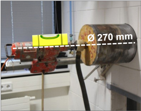
Fig. 2 – core hole drilling
