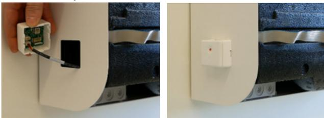
Reinstall the ventilation unit according to the respective installation instructions. Then restore the power supply and perform a function test.
